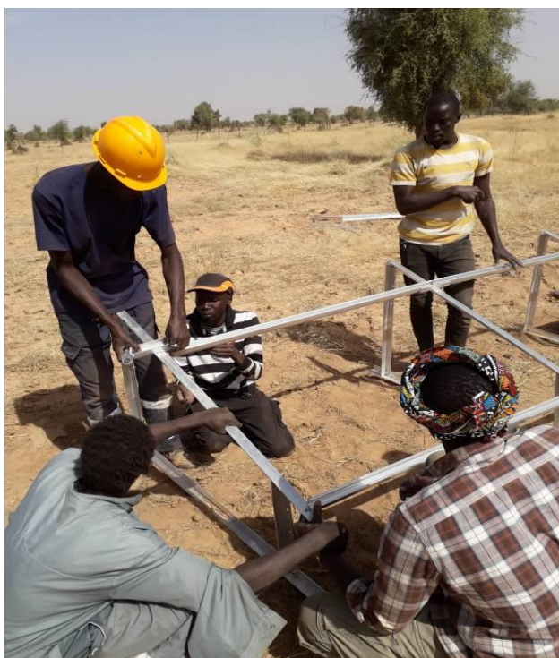
Photo1 montage support panneaux
